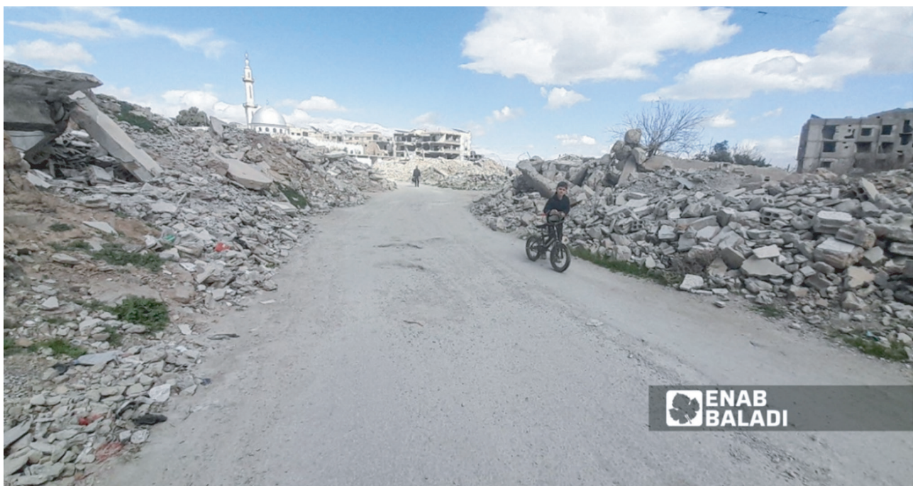
Figure 6: Building Rubble in Qaboun, Damascus
